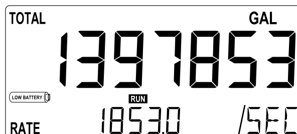
Fig. 4: Example of low-battery alarm.
